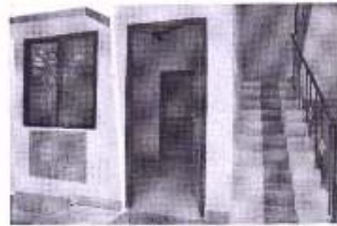
Exterior finish of GFRG panels
