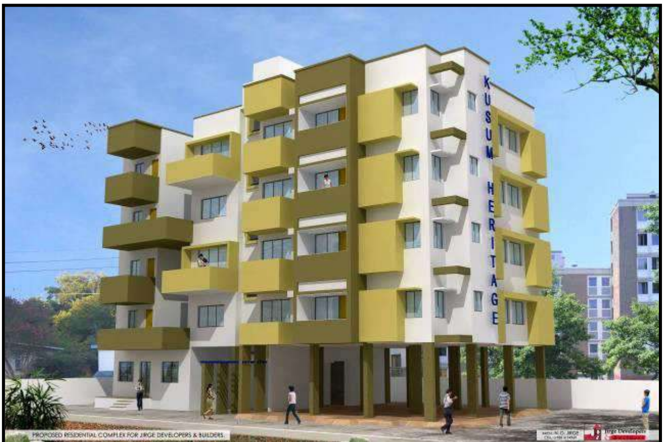
A.K. Builders Himmat Bahadur Parisar Kolhapur, 2007
