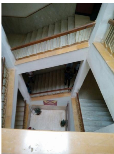
Centrally located Staircase
